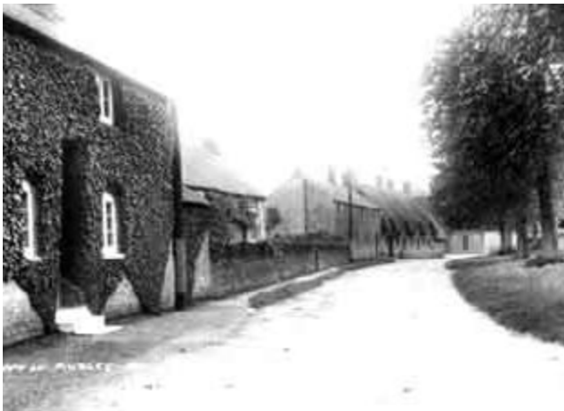
The Garden House with The Cottages in the distance, Cherry Street.
